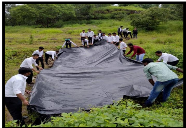
Finishing the laying of plastic at the bottom of the pond
