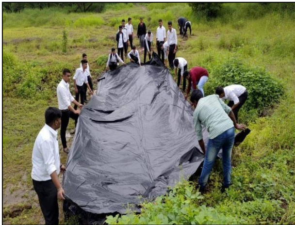
Creating artificial pond for water storage
