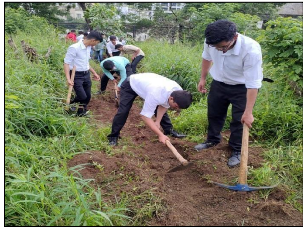
Ploughing the path for water stream
