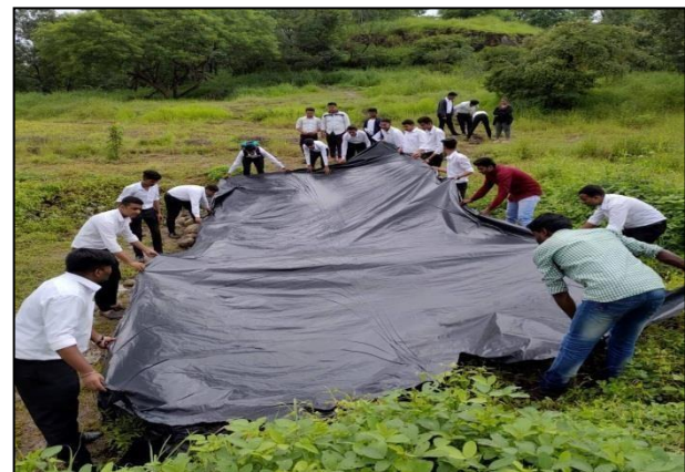
Finishing the laying of plastic at the bottom of the
